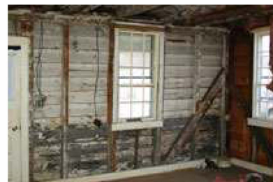
Early interior finishes
